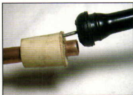
You might have to carve away part of the valve so it fits next to the copper.
