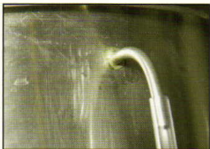
A close-up of the silver brazed fitting. Brazing uses a filler metal to join two metal surfaces together.
