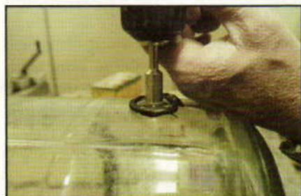
Keep the reservoir full of water to keep the bit cool as it cuts the glass. Excess heat would crack the glass.
