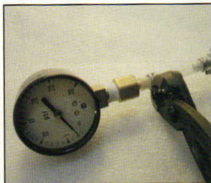
The final step is to crimp the Oeticker clamps to hold the tubing.
