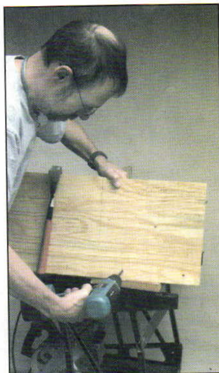
Predrilling depressions for screw heads (countersinking) insures tight joints and a smooth, snag-free surface.
