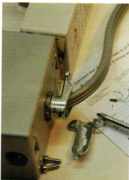
Thread the cable through the box and into the controller. A bottom connection was preferable for my brewhouse.
