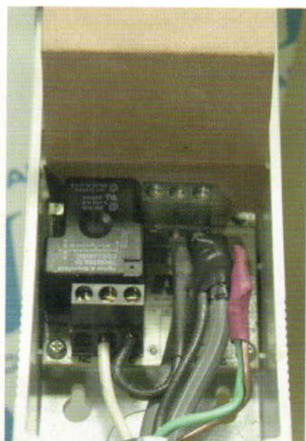
Note that the green and bare copper grounds have been joined and partly covered with heat-shrink tubing.
