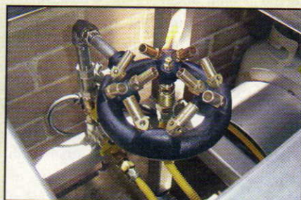
Picture 7: The pilot-light driven low pressure burners are temperature switch controlled and fire only when necessary.
