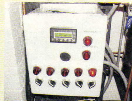
A view of the control panel that has the multi channel temperature controller and on/off switches for the heating elements and pump.
