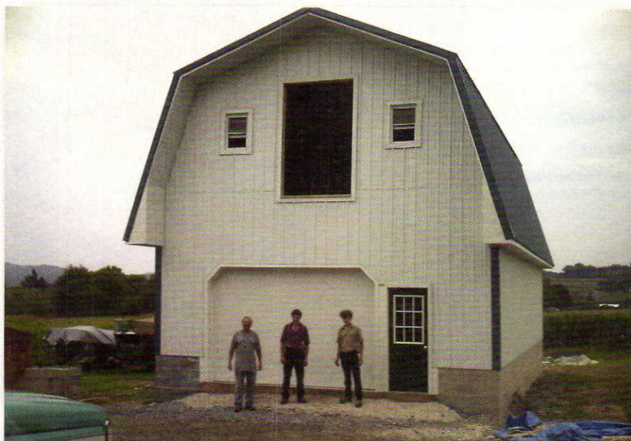
A garage fire destroyed Mike Knaub's garage, which housed all of his homebrewing equipment. In its place, he built this new structure that he calls the Phoenix Brewery.
