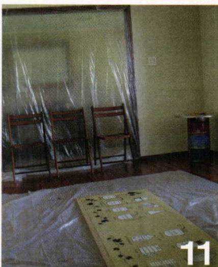
A makeshift clean room was prepared for applying epoxy to the bar top.
