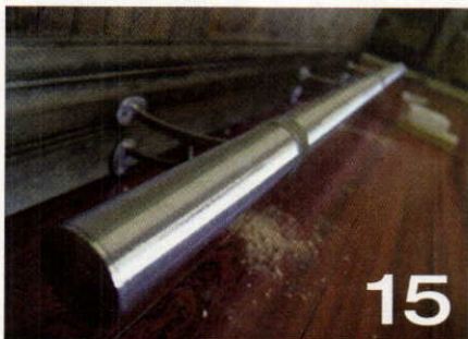
A stainless steel footrest is screwed into the frame 2x4s for adequate support.
