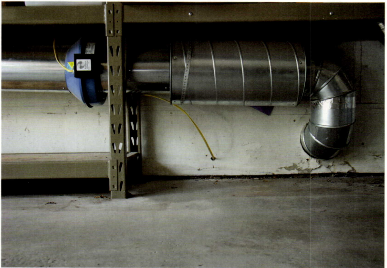
Ventilation duct with a fan (in blue) and a silencer (the widened area to the right of the fan) to reduce noise. Airflow is from right to left (through the silencer, then the fan).
