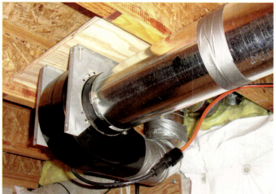
Ventilation is required indoors to remove evaporating water, heat and combustion gasses from the burner, not to mention aromas. Ductwork from Al Feeberg's brewery shown.
