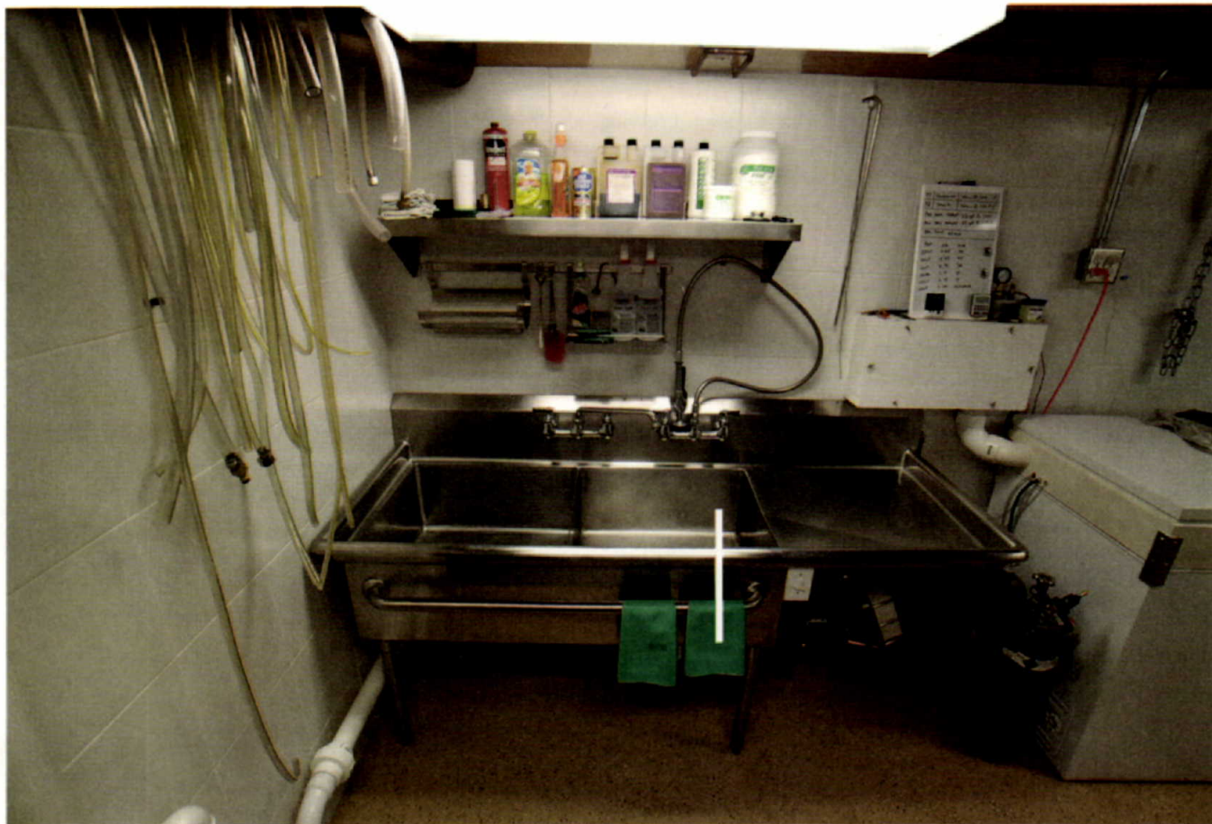
A large stainless steel sink with a sideboard is ideal for cleaning brewing equipment, especially the bulkier vessels, and for letting vessels and equipment dry. You will never be sorry for allocating adequate space for a good sink.
