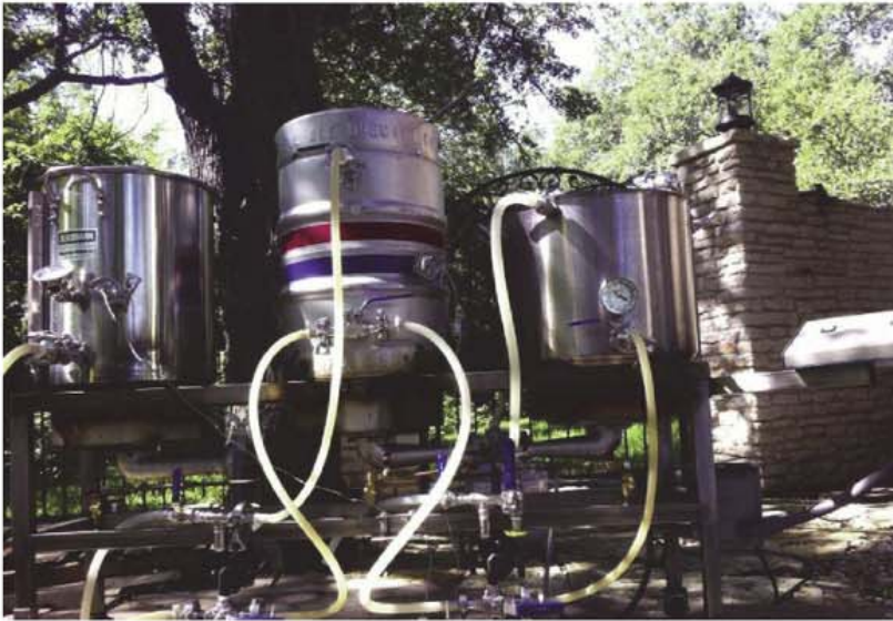
With two well-positioned pumps and 3-way ball valves connected to an all-grain system, a homebrewer can move all of the brewing liquid in a batch of beer from start to finish.
